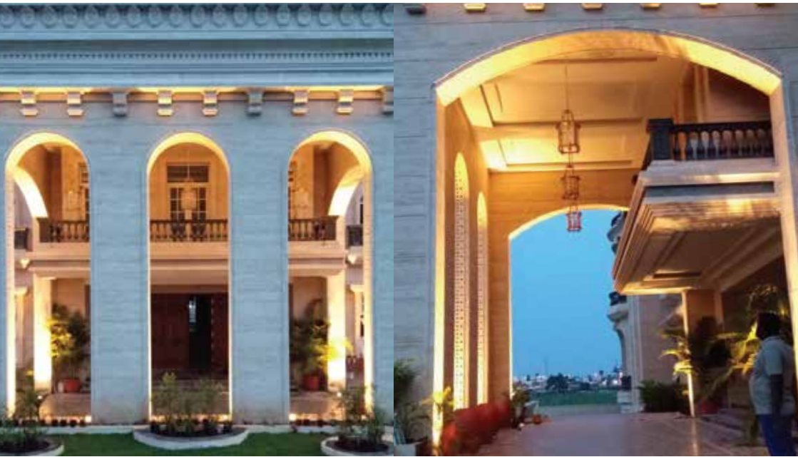
PRIVATE RESIDENCE, CHENNAI
