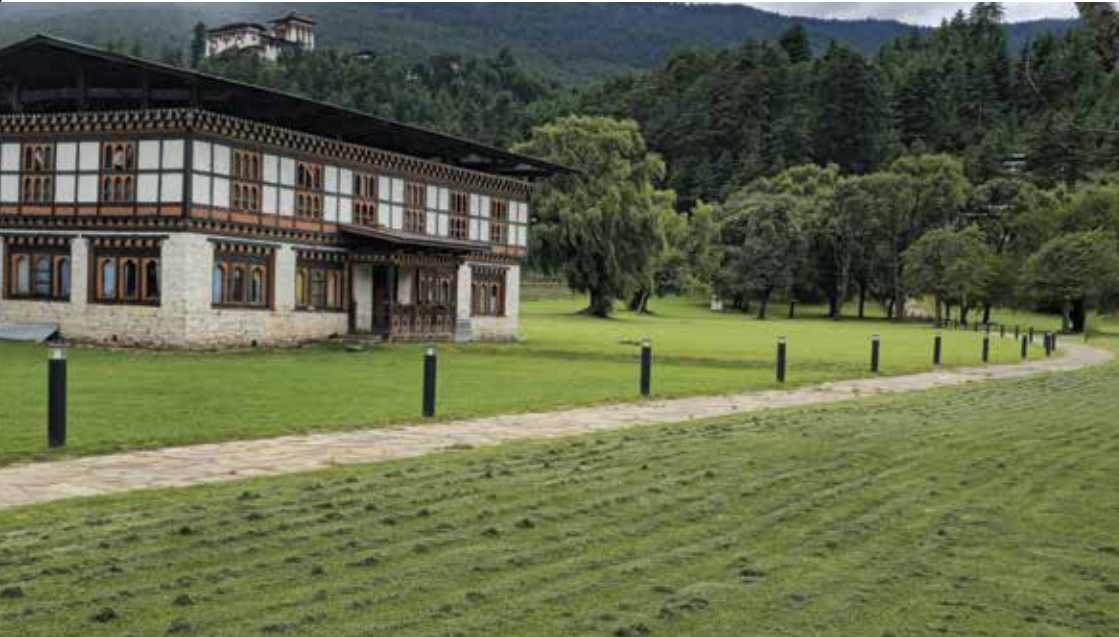
WANG PALACE, BUMTHANG, BHUTAN
